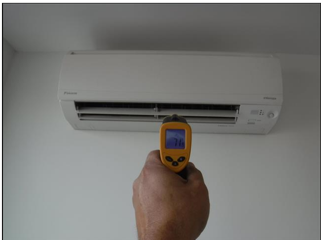
3.0 Item 1(Picture) heating register
