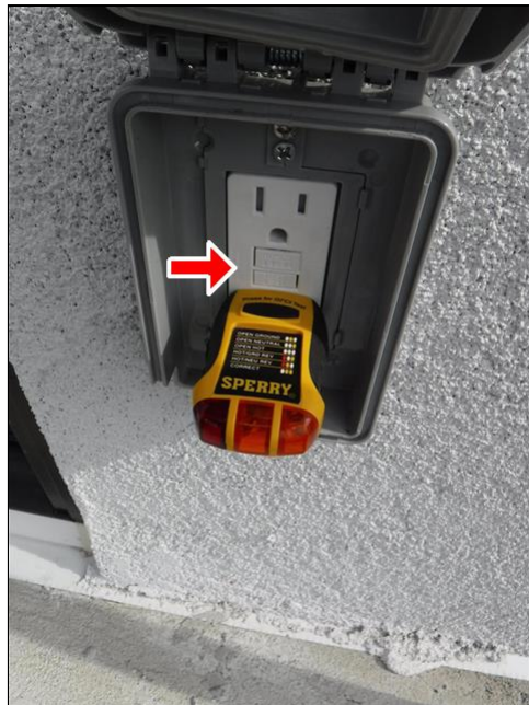
5.2 Item 2(Picture) balcony area off master bedroom
