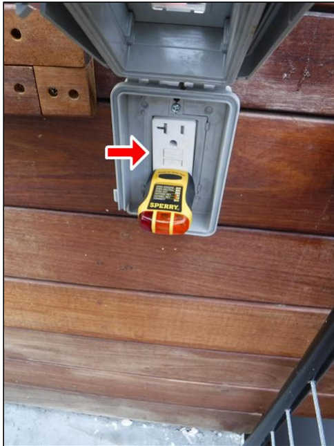
5.2 Item 1(Picture) front exterior of building
