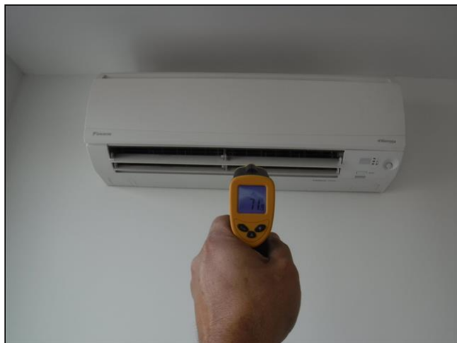
3.0 Item 1(Picture) heating register
