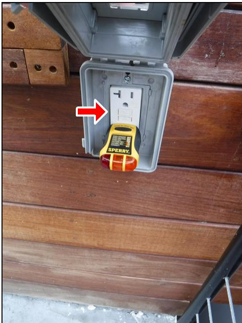
5.2 Item 1(Picture) front exterior of building
