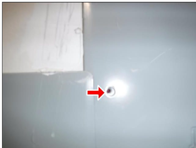
5.0 Item 2(Picture) main panel in basement
