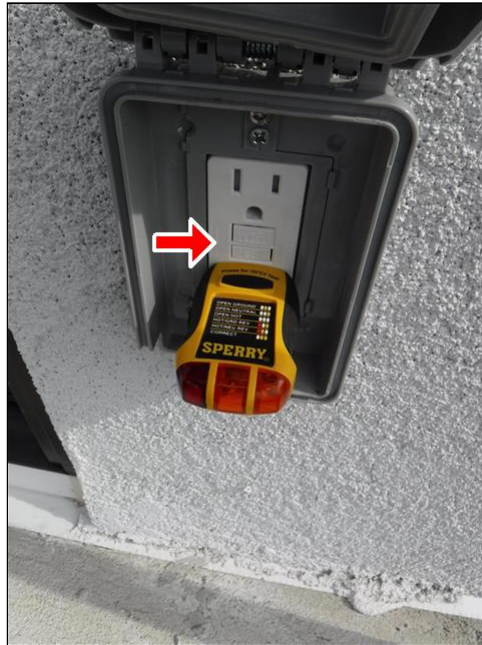
5.2 Item 2(Picture) balcony area off master bedroom
