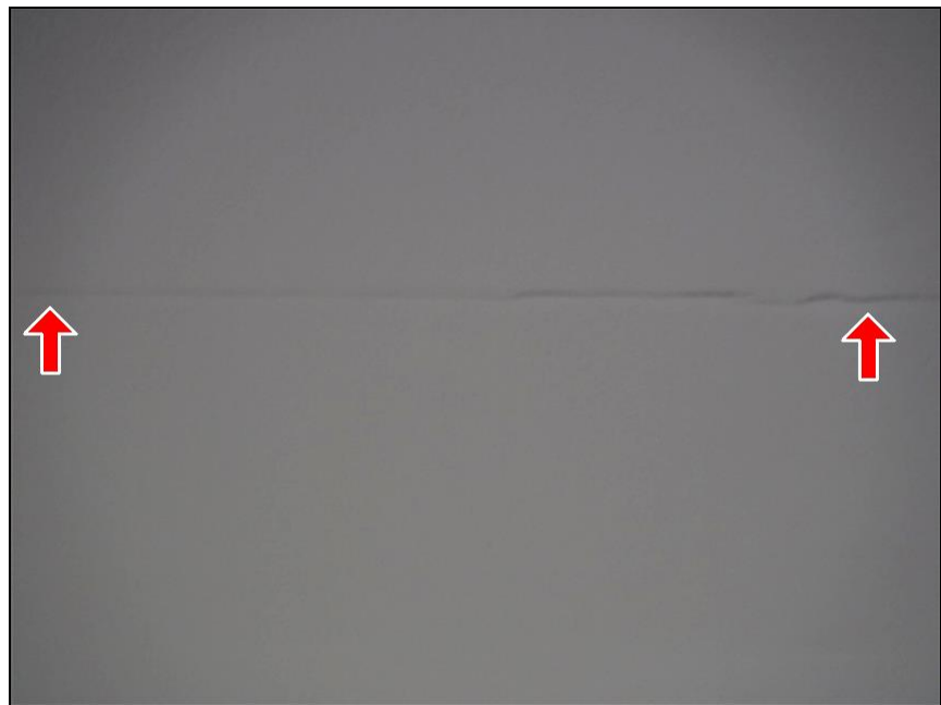
8.0 Item 1(Picture) seam showing on ceiling
