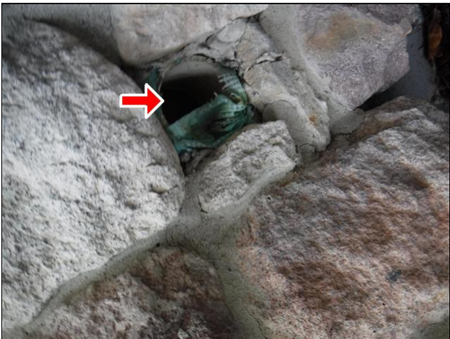
2.2 Item 14(Picture) waste line vent cover missing
