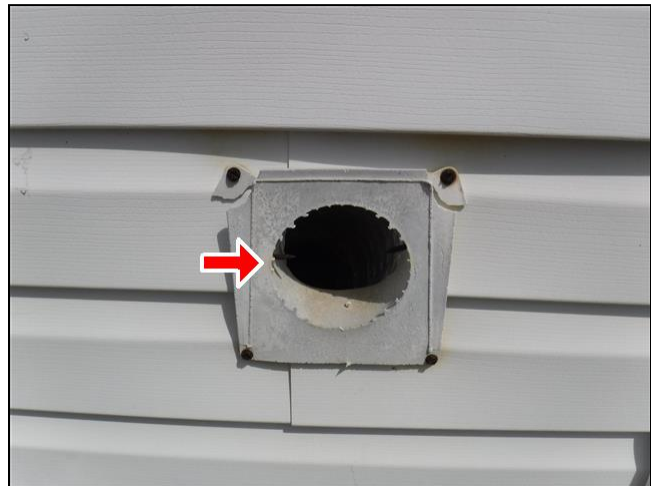
2.2 Item 13(Picture) dryer vent cover missing
