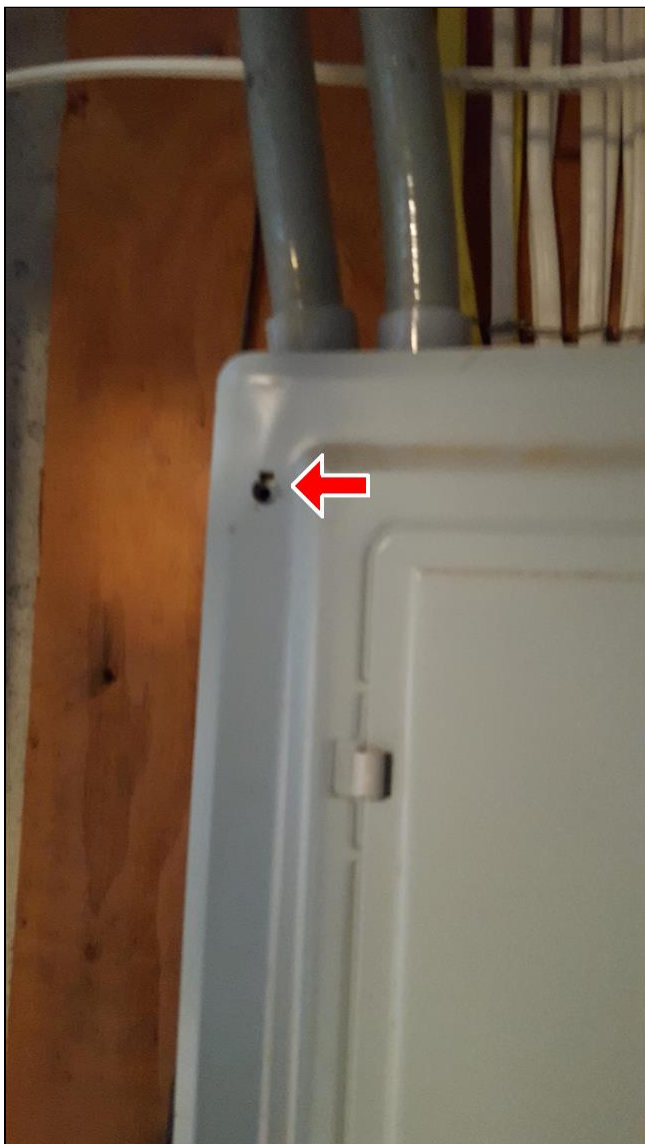
6.1 Item 2(Picture) screws missing at panel
