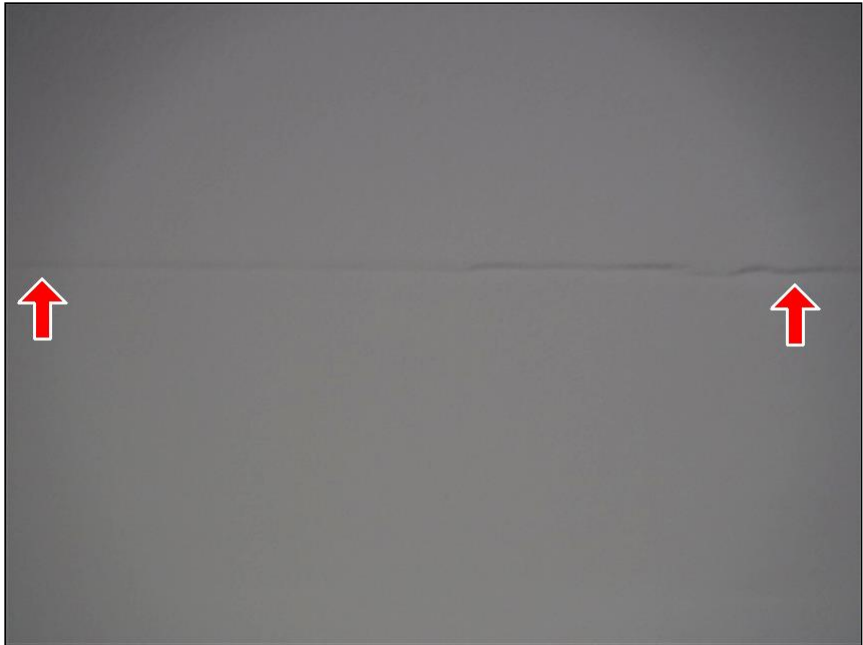
8.0 Item 1(Picture) seam showing on ceiling
