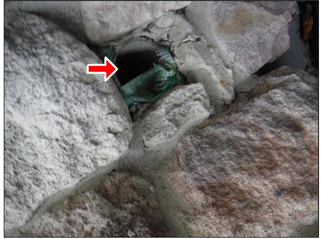
2.2 Item 14(Picture) waste line vent cover missing
