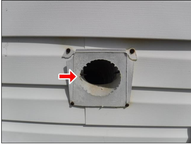
2.2 Item 13(Picture) dryer vent cover missing
