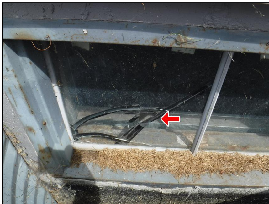
2.1 Item 5(Picture) basement window broken
