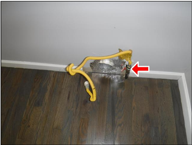
gas line for dryer
