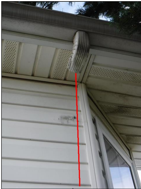
1.2 Item 2(Picture) gutter missing downspout
