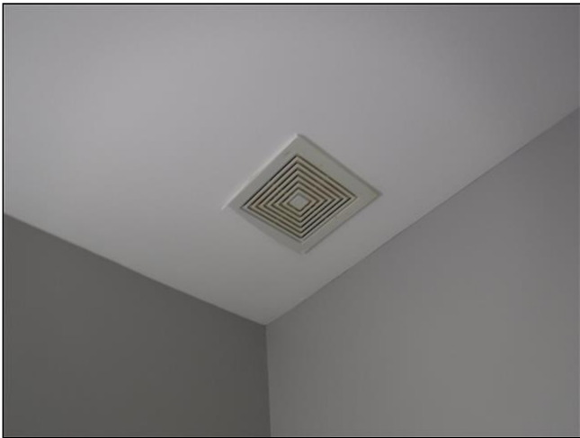
bathroom exhaust
