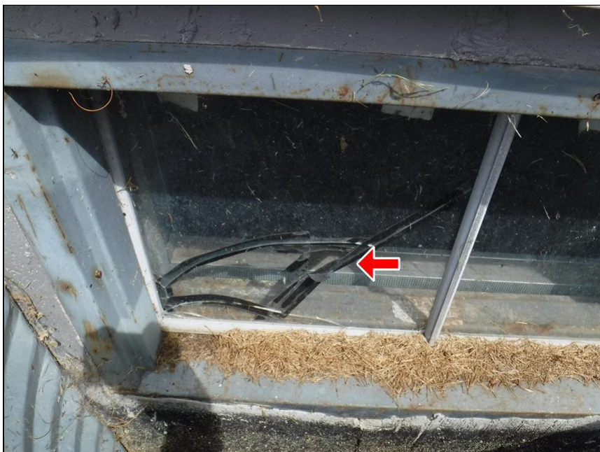
2.1 Item 5(Picture) basement window broken
