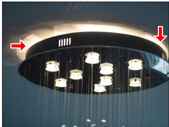
6.3 Item 8(Picture) loose lighting fixture
