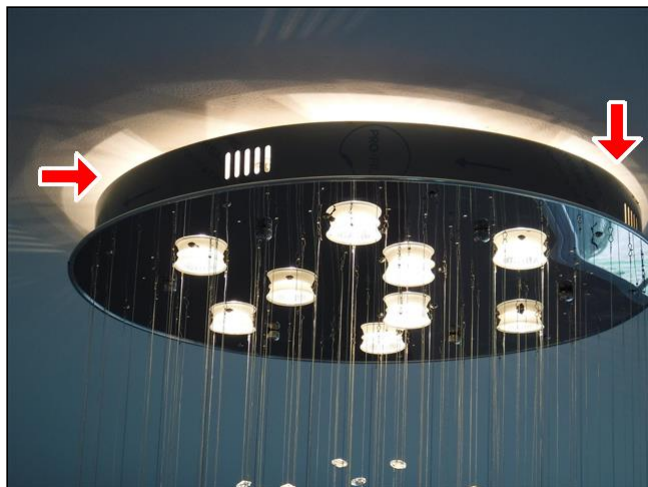
6.3 Item 8(Picture) loose lighting fixture
