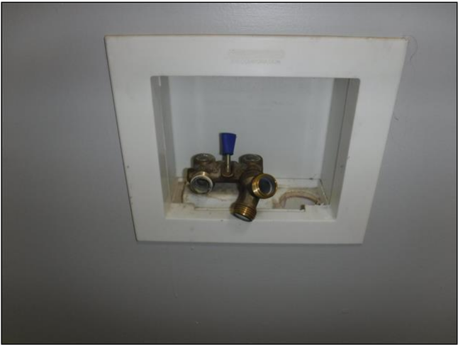
water supply to washermachine
