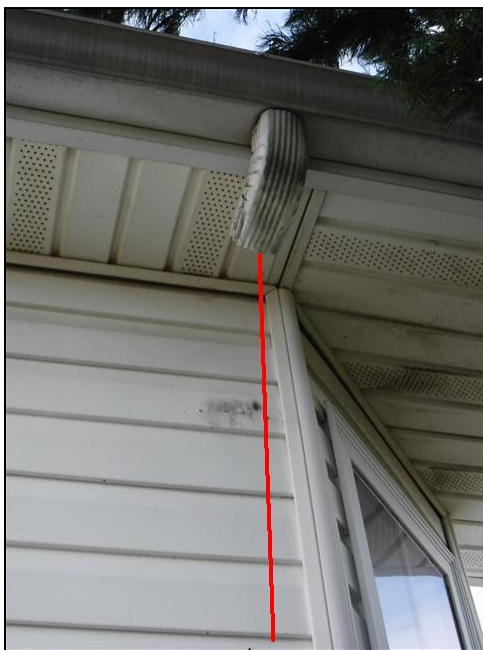
1.2 Item 2(Picture) gutter missing downspout
